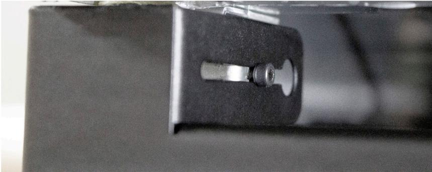
6. Adjust grille depth and tighten both adjusting screws with Allen wrench.
